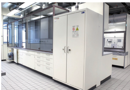
Vacuum supply of a laboratory line with safety exhaust hoods
