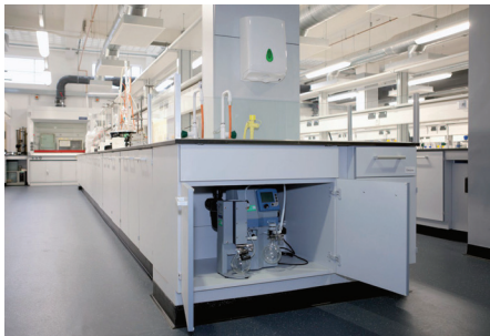
One pump - many users: network installation with Peltronic cooling without water connection for solvent recovery
