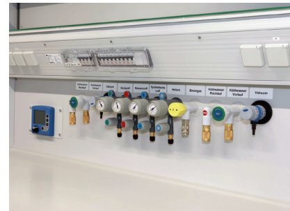
Controller installation within the media column
